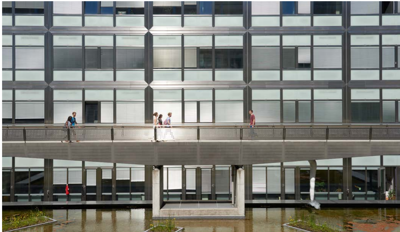
Excellent infrastructure is a central factor in the success of ETH Zurich. Strategic real estate planning requires the anticipation of academic developments (example: the HCI building, which is used for the departments of Chemistry, Biology and Materials Science).
